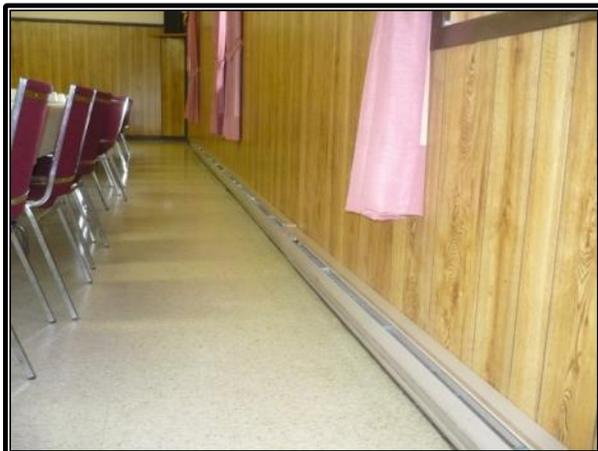
View of typical electric baseboard heaters located within Site Building B.
