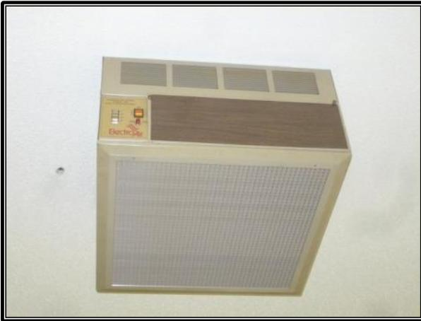
View of an electronic air cleaner located in the ceiling of Site Building B.
